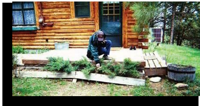
Flammable vegetation in direct contact with
