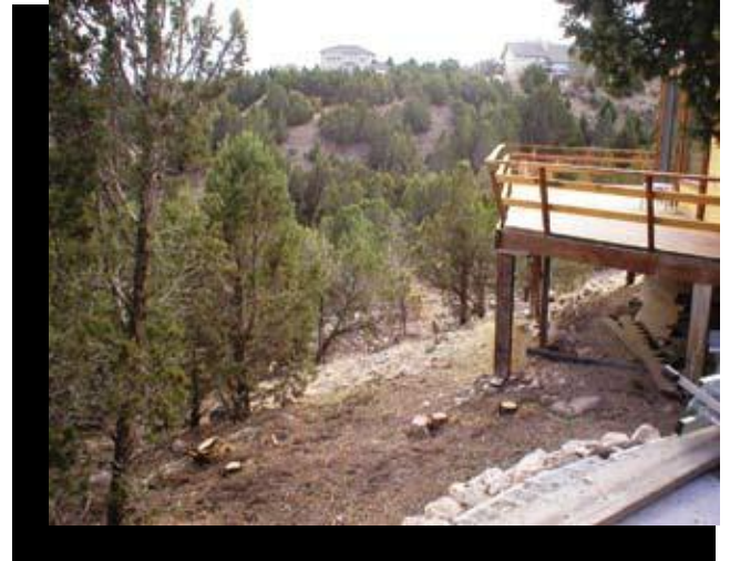
After mitigation work, deck is less likely to ignite
