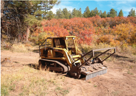
Figure 4: Mechanical treatment using a timberaxe.
